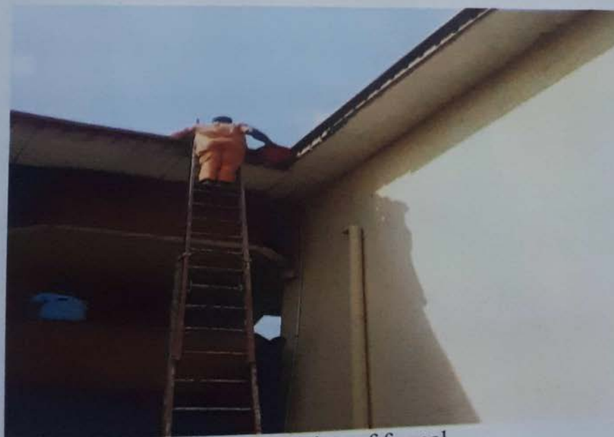
Fig. 3.2 Fixing of funnel
