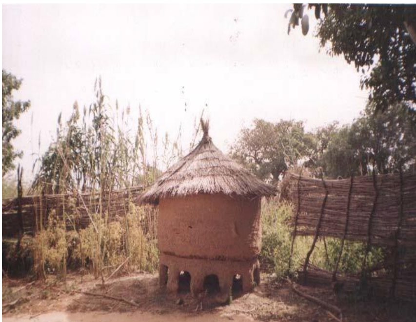
Plate 1: Mud Rhombus with stone grillage foundation floor assembly and thatched roof at Ibiense
