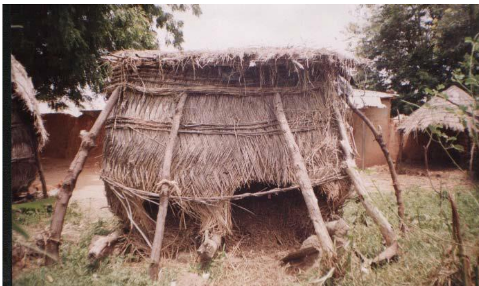
Plate 3: Failed Thatched Rhombus after 8 years of use at Jattu
